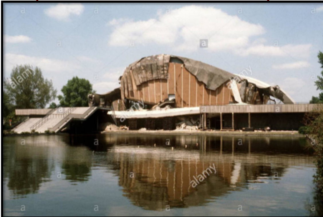
Hydrogen intake causing collapse of roof
