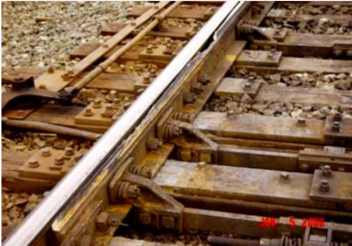
Severely worn switch blade
